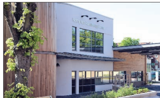
The Nottingham Radiotherapy Centre is a recent example of the direction the Trust is taking in renewing its infrastructure to a low carbon standard. This building was designed to comply with a 'BREEAM Excellent' standard and incorporates a number of sustainable technologies.
